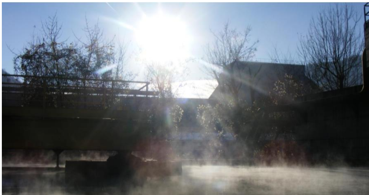
Wastewater treatment plant and fume aspiration system
